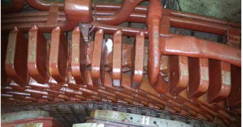
Fig. 13 Rebuilding of Stator-winding
