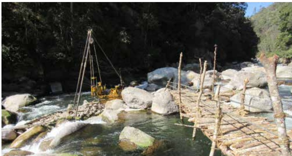
Fig. 12 Additional Investigation Works at Dam Site
