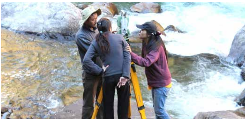
Fig. 11 River Survey Work in Progress at Nyera Amari HPP Site below Thungkhar Village
