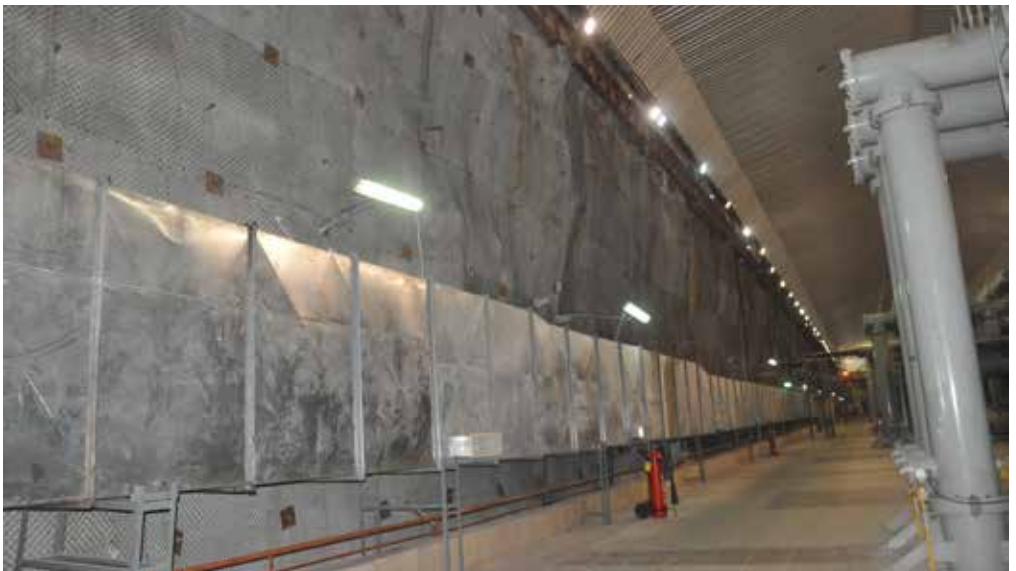
Fig. 14 Remedial Safety Measures Adopted for Failing Rock Bolts in the Powerhouse
