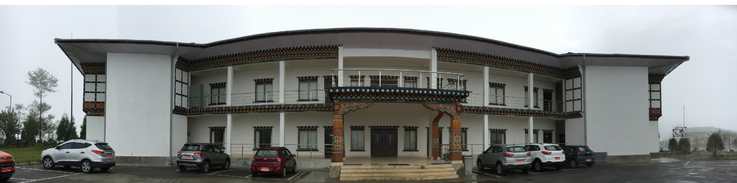
HRDC office at Rinchentse
