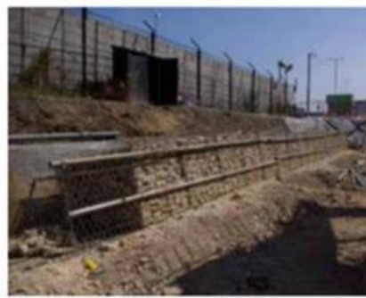
b) Use of pipes
