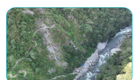
2023 Feasibility Study of 90 MW Jomori Hydropower Project
