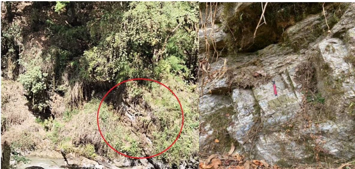
Photo 4-2: Rock exposure at right bank 10m d/s of weir axis (left) and at intake area (right)
