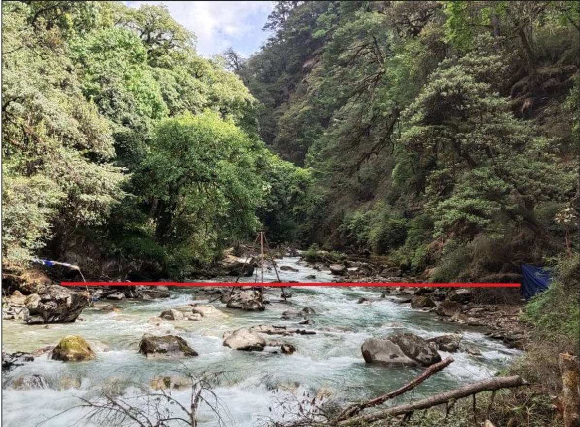
Photo 4-1: Location of weir axis
