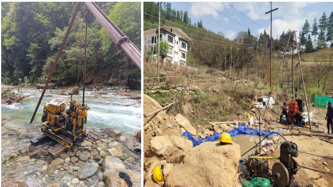
Photo 4-11: Core Drilling at Intake and Power House
