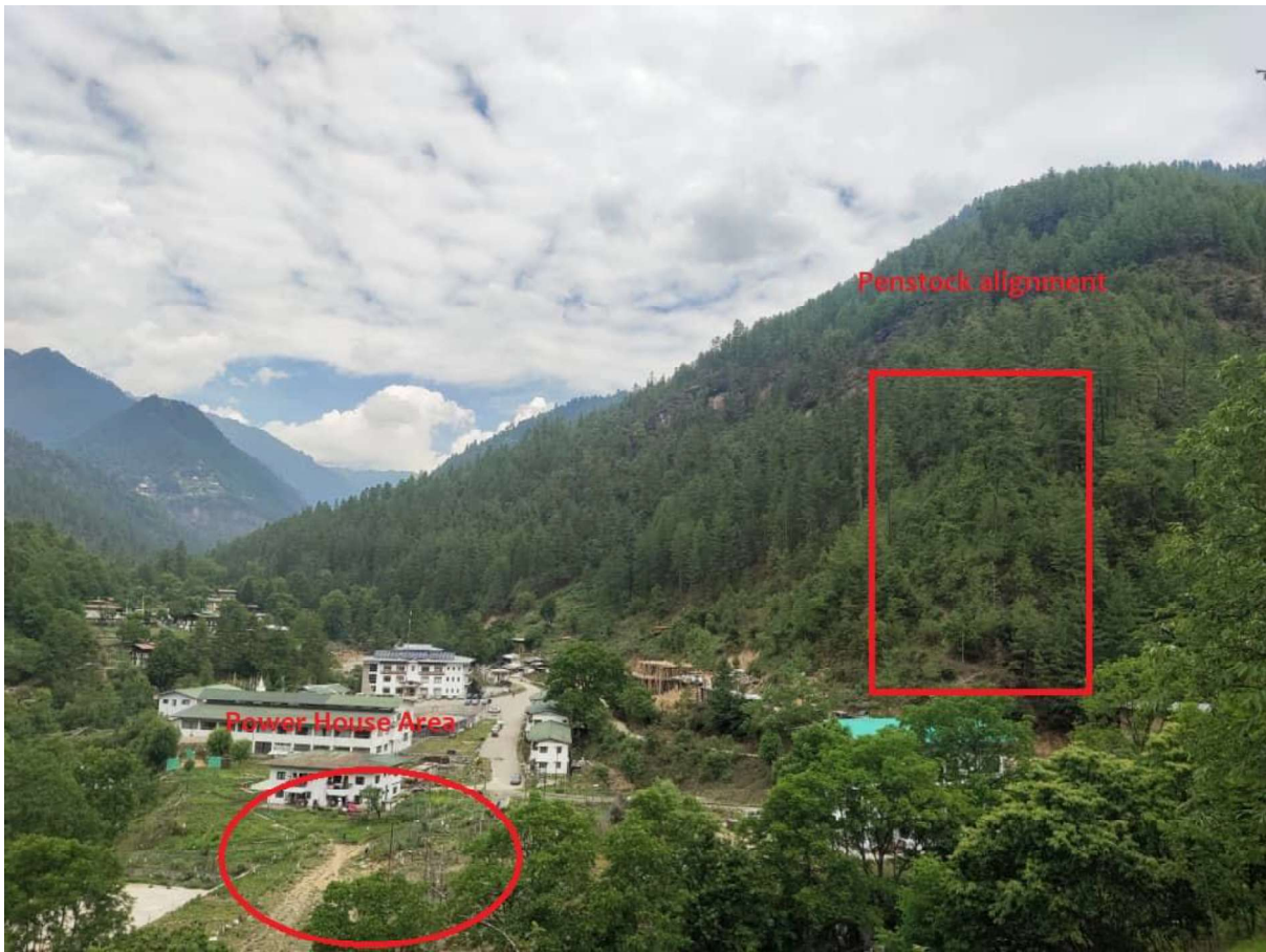
Photo 4-12: Penstock and Power House Locations
