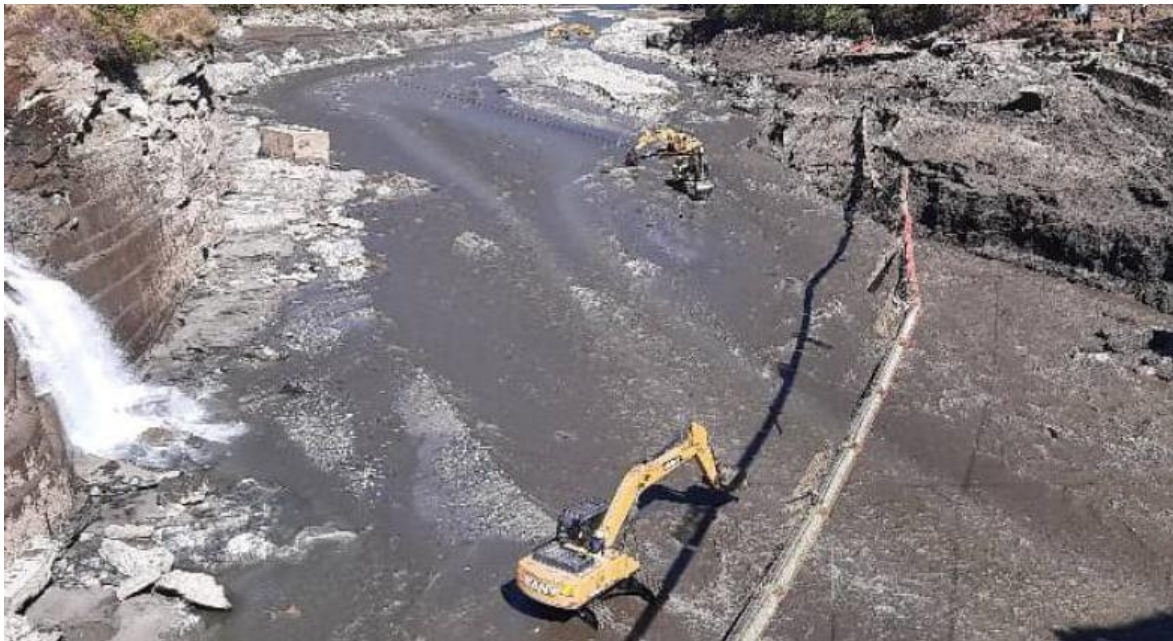
Figure 5-10: Sediment dredging at the Chucka Reservoir
